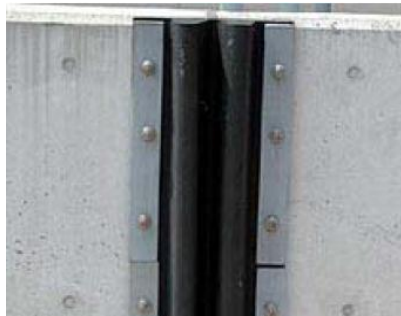
Figure 10-6 Gap with flexible material
