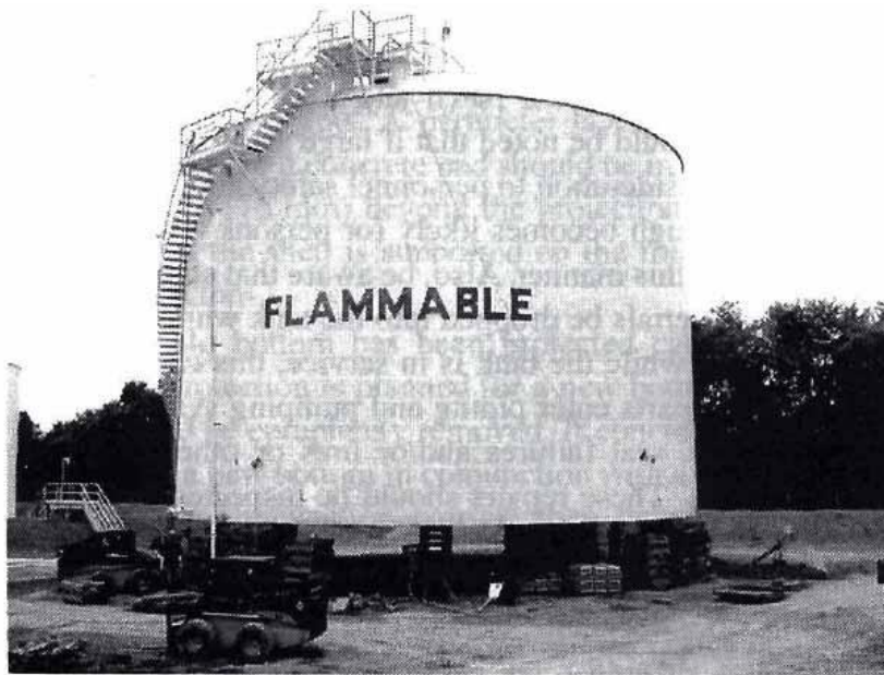
Figure 6-19 Lifted tank to repair below layer
