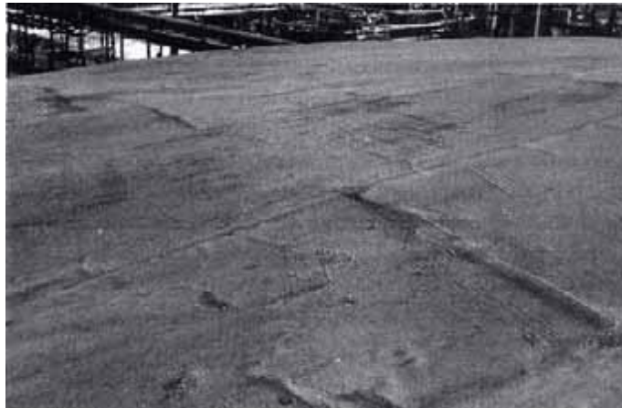
Figure 6-28 bitumen roof coverage
