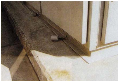
Fig. 9-6 Movement of room unit
