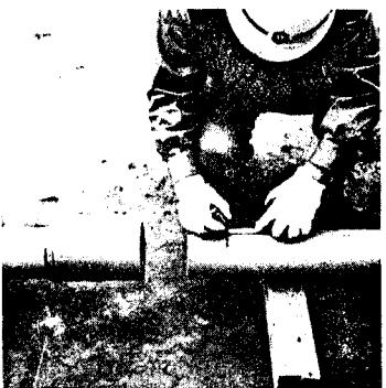
\* Checking the zero point and marking the engagement length
