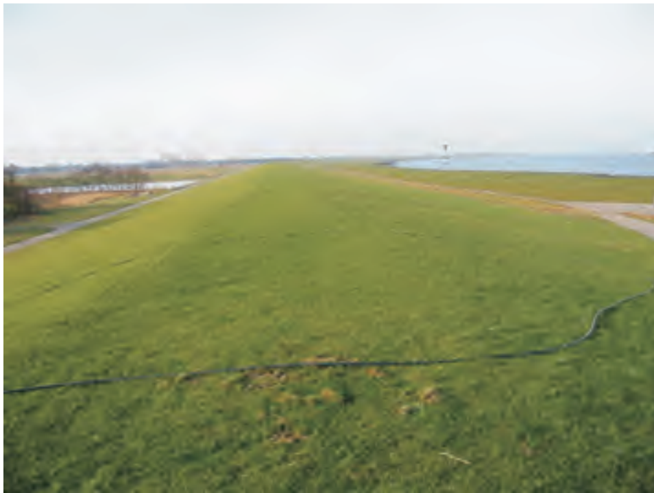
Fig. 5.15: Dike covered by grass (photo: SCHÜTTRUMPF)
