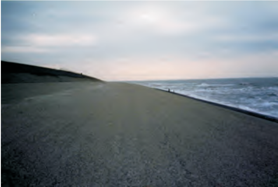
Fig. 5.16: Dike covered by asphalt (photo: SCHÜTTRUMPF)
