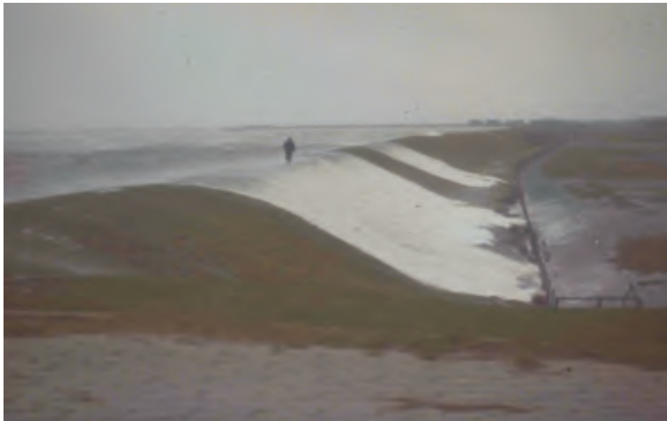
Fig. 5.33: Wave overtopping on the landward side of a seabed (photo: ZITSCHER)
