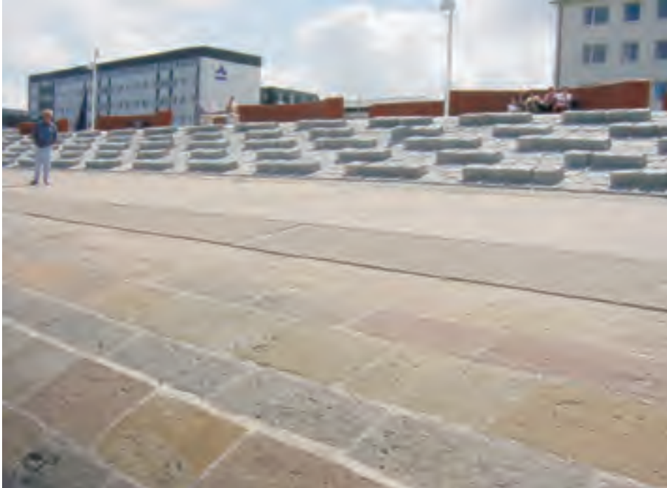
Fig. 5.19: Example for roughness elements (photo: SCHÜTTRUMPF)
