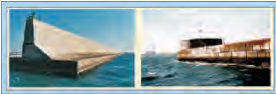
Fig. 7.1: Examples of vertical breakwaters: (left) modern concrete caisson and (right) older structure constructed from concrete blocks
