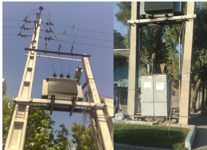
Figure 5-14: Distribution supports and aerial transformer
