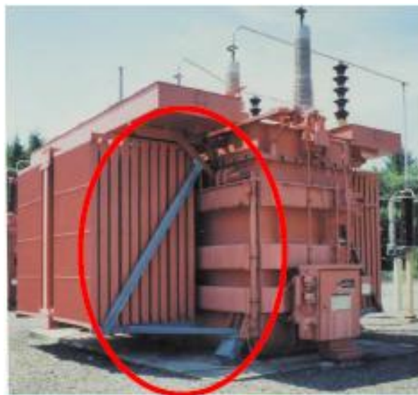
Figure 5-5: Reinforcing bracing of transformer's radiator
