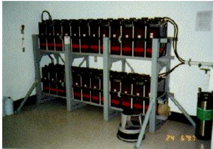
Figure 5-10: Batteries shelf bracing for controlling overturn
