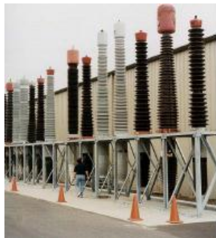
Figure 5-12: Bracing spare equipments in warehouse
