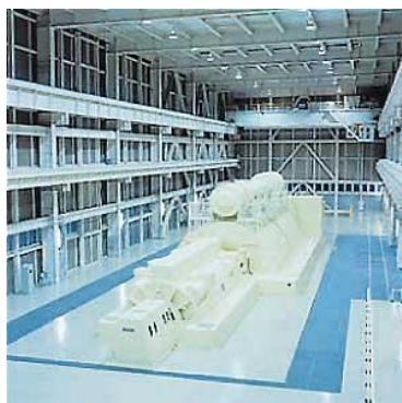
Figure 5-2: Steam Turbine
